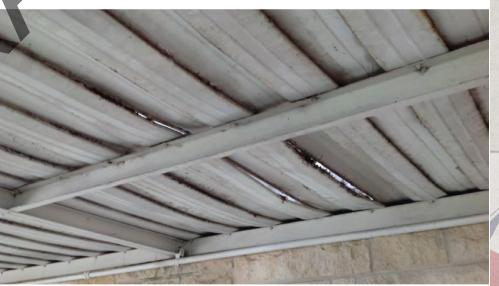
Figure 8-1. The Canopy around the Golf Course Club House. You can see the deterioration and damage that has happened due to weathering.
